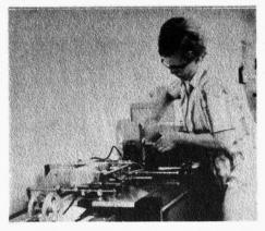
The Scriptomatic machine automatically addresses the order forms. These addresses are positioned so they will be visible through the clear window in the catalog envelope when they are inserted. The addressing machine is capable of handling 6,000 address cards an hour.
